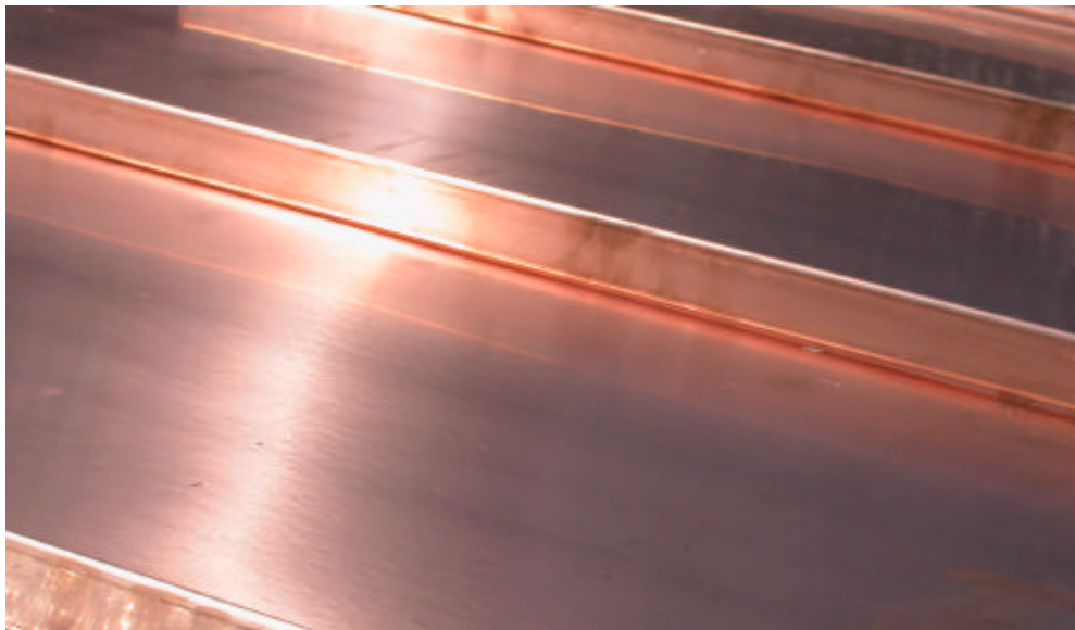
Astro Copper Roof detail
